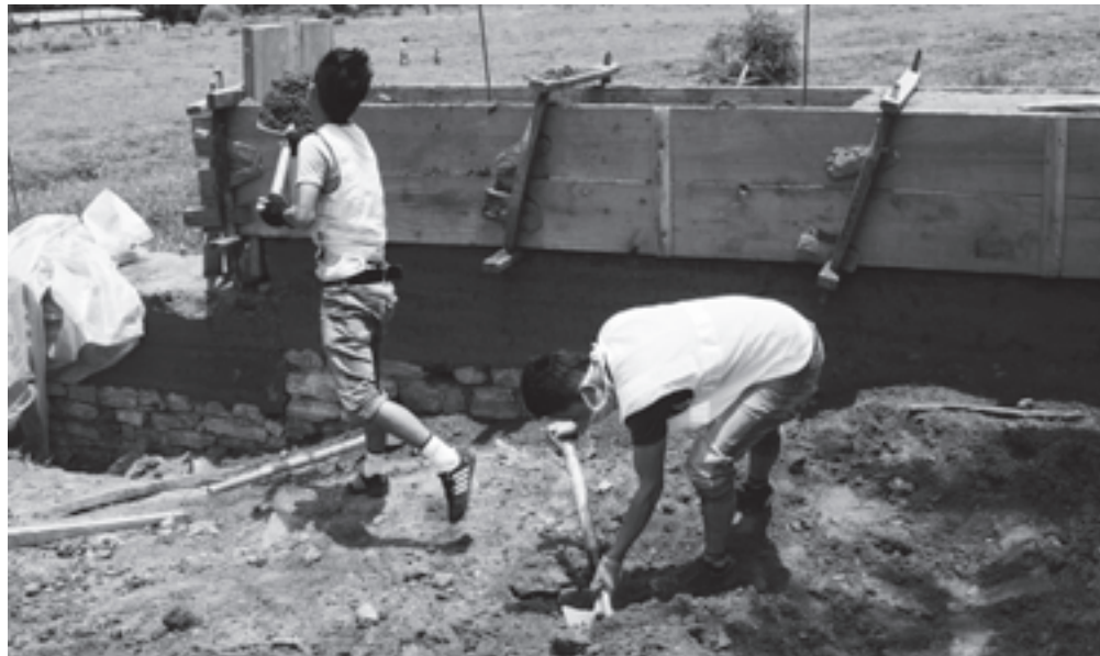
VTI graduates build a mud wall in Thimphu (File photo)
