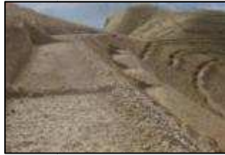
Photo: Level terraces
