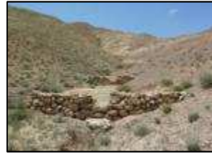
Photo: Check dams
