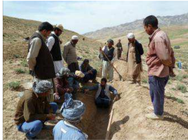
Photo: Technical guidance by GS project manager
