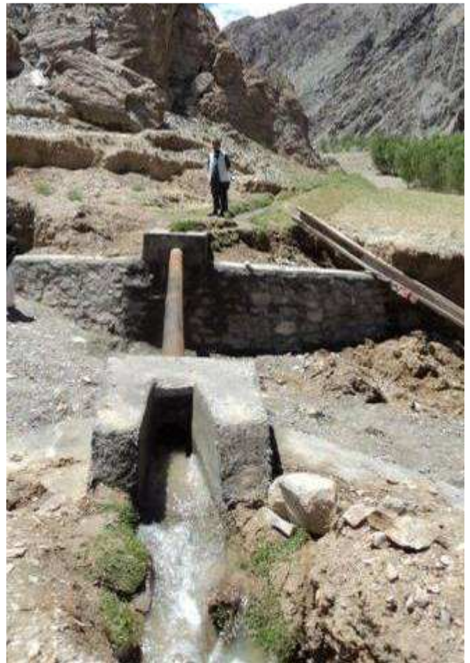
Photo: An aqueduct constructed in Saighan is benefiting 60 families by supplying uninterrupted irrigation. Communities contributed 20% of the project cost.
