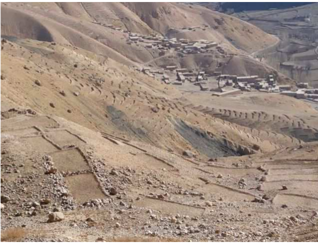
Photo: Watershed management measures (terraces and contour trench) have been applied on a large scale in Ruy-i Doab.
