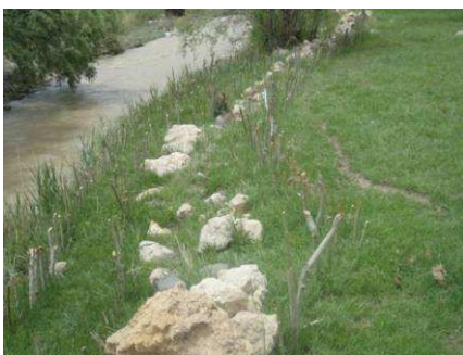
Photo: Tree cutting planted along streams for bank stabilization.
