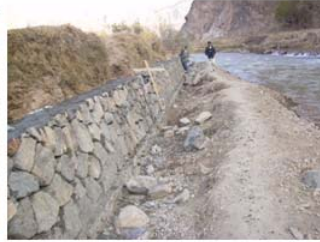
Construction of protection wall
