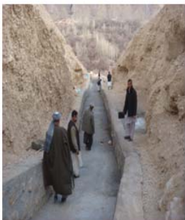
Construction of flood way
