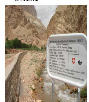
Completion of protection wall
