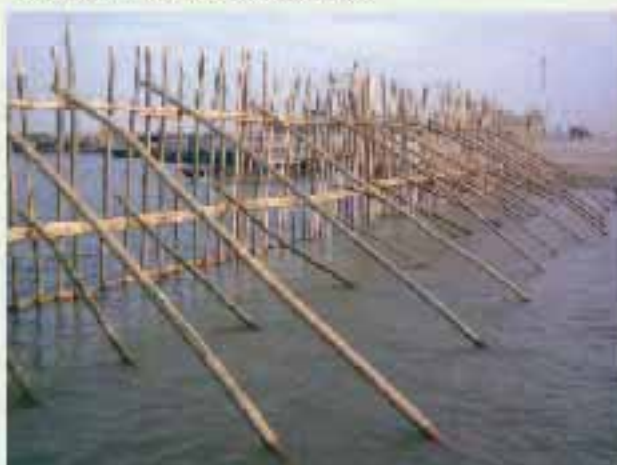
Photos 4,5 : Bandel and pilling against river erosion
