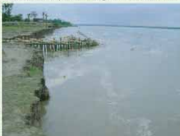
Photo 3 : Hati protection against wave erosion
