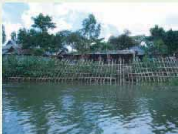
Photo 3 : Hati protection against wave erosion
