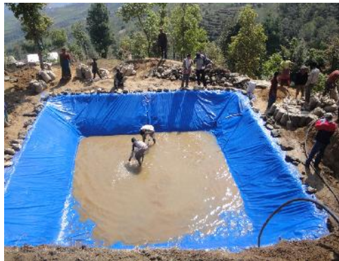
Figure 2: Excavated Pond with Silpaulin Lined
