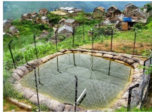
Figure 3: Pond with Soil Cement Jut bag lining
