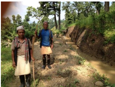
Two maintenance workers on a cleaned canal in Jhilmile Talbari Irrigation Scheme, Surkhet
